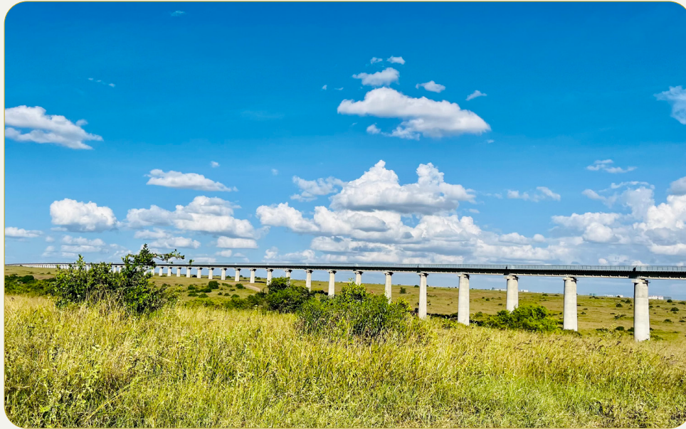
Nairobi National Park, underpass for Wildlife, for railway: Nairobi-Mombasa
