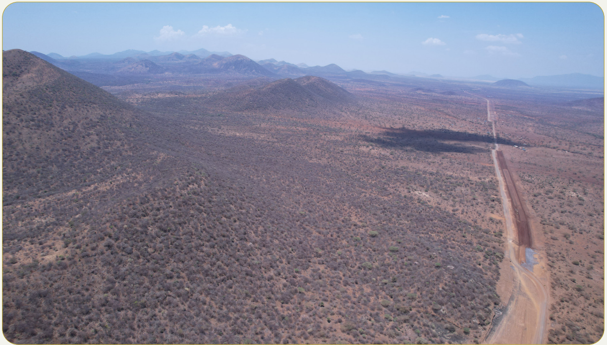
Yaq-Barsadi Village: The Road Section
